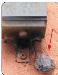
Corrugated pipe entry protection
