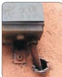
Corrugated pipe entry protection
